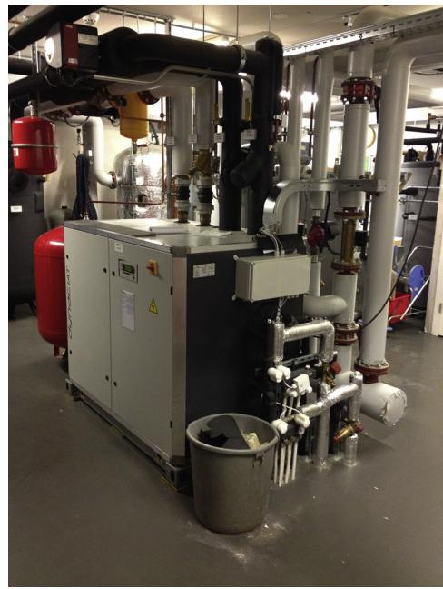
**Fig. 4.** A large-scale heat pump installation in the basement of one of the premises of Habion. The design of sustainable energy systems in the built environment also includes having sufficient space available for the placement of technological equipment.
