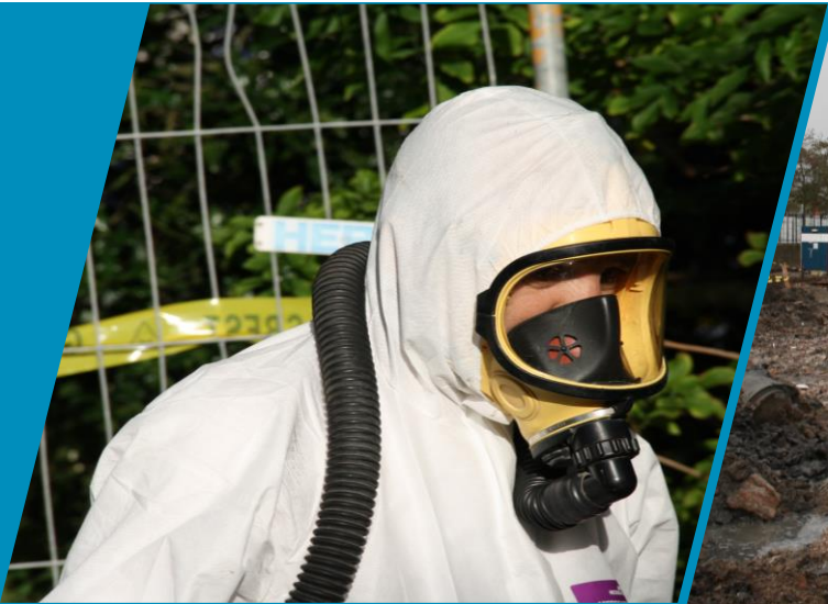
Asbest/ Chroom-6 sanering
